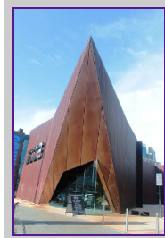
Fig. 10 Australian Centre for Contemporary Art , Ingresso forma monolitica.
